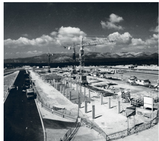
Building the Paul-Ricard circuit
