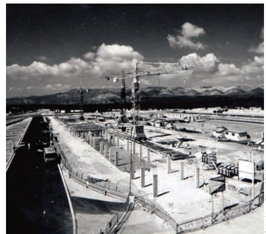
Construction of the Paul Ricard circuit
